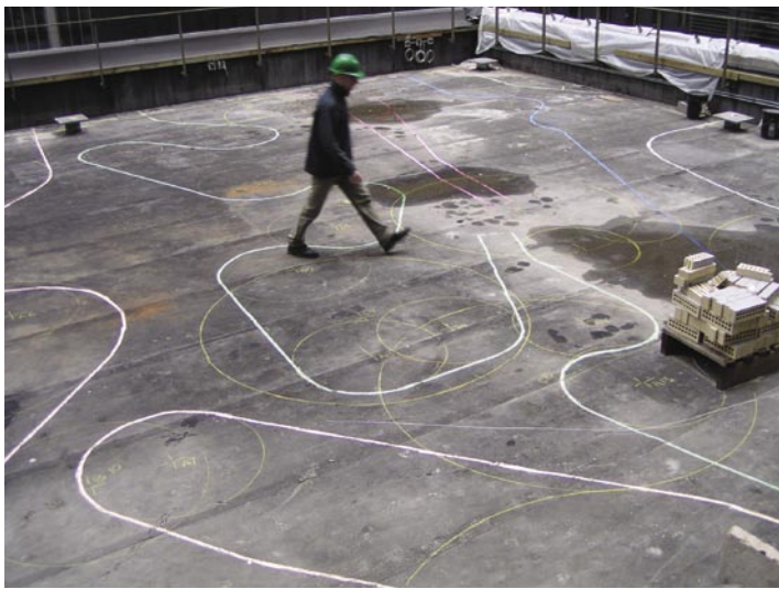
Mock-up of roof garden layout, January 2004
