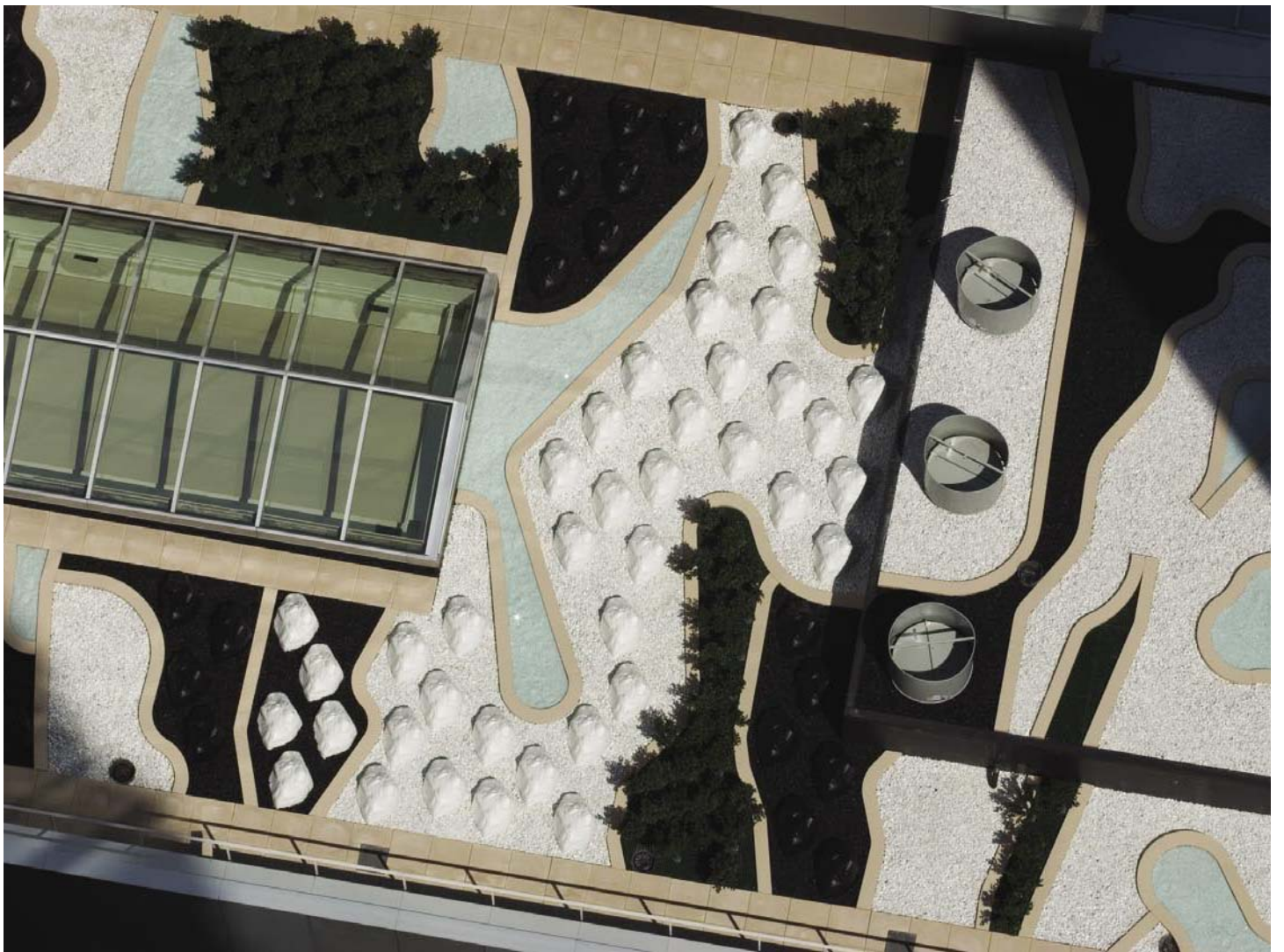
South roof, view from 40 West 53rd Street
